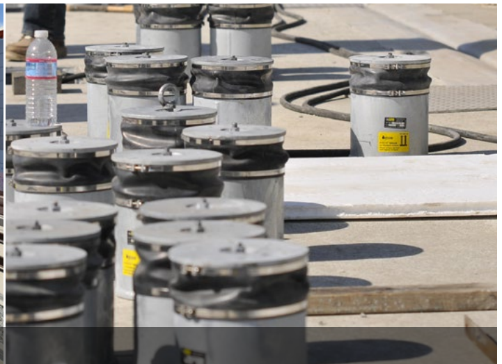
Floating Slab Track (FST) / EBS System, Expo Line, Los Angeles, USA
