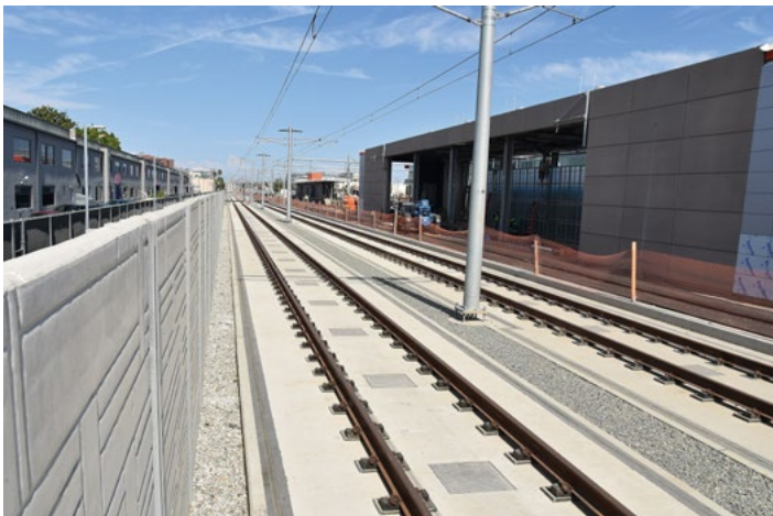
Floating Slab Track (FST) / EBS System, Expo Line, Los Angeles, USA
